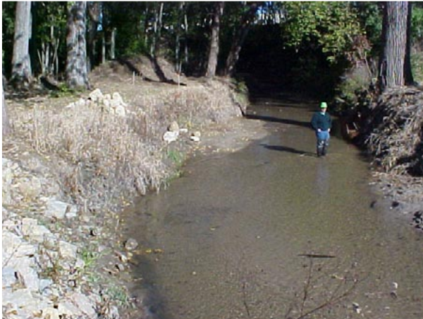
The Pheasant Branch stabilization project
