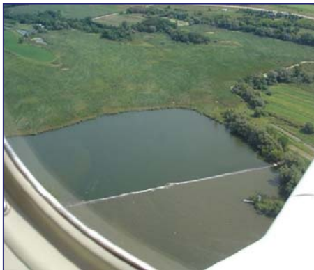
Aerial photograph of Geotube breakwater structure on Lake Sinissippi.
