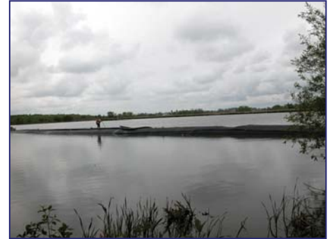
Sediment-filled Geotube breakwater structure on Lake Sinissippi.
