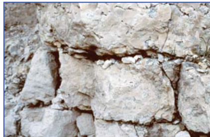
Typical cracks in limestone bedrock, allow surface water to move quickly down to our groundwater without filtering of nutrients, pathogens or other waste products.
